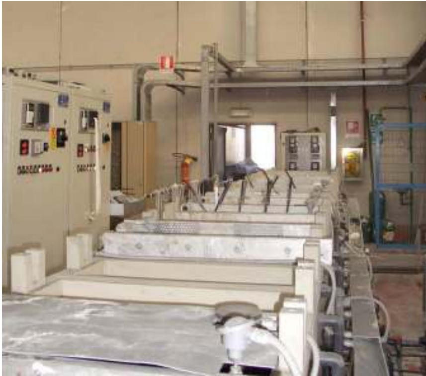
Figure 25 – Multi-purpose pilot line in Italfinish
